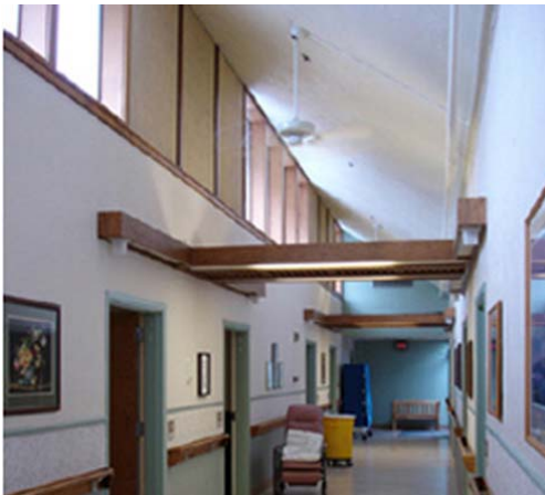
Figure II: The diffused daylight coming into this corridor creates a pleasant visual environment along with the spectrum and higher light levels for circadian rhythm.
