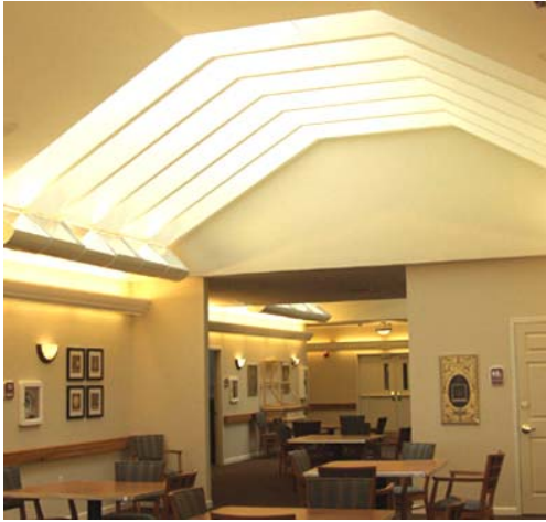
Figure IV: This is the same facility with large skylights added to the dining and activity areas, increasing the daylight fenestrations by 320 percent.
